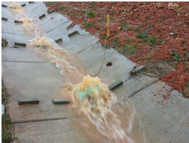
Figure 3-9: A stream inflow where a 703d#3 Floc Log was placed on a concrete ditch.
