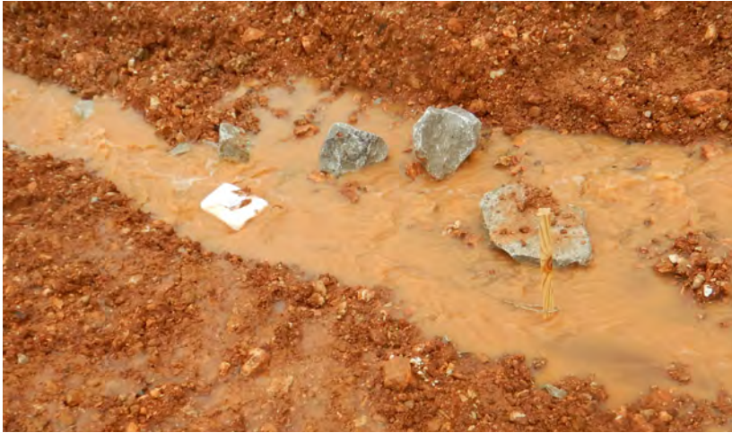
Figure 2-8: Photograph of the APS 703d type Floc Log roped around a stake. Photo taken by Bryan Signorelli (AHTD) on June 18, 2015.
