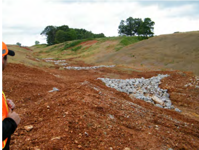
Figure 3-8: Photograph of the site chosen for the first field test. One inflow stream was from the left side of the photo, which enters the small and shallow basin. A second inflow stream is pictured in the background, which included a series of small basins with intermittent rock checks. Photo taken by Bryan Signorelli (AHTD) on June 18, 2015.
